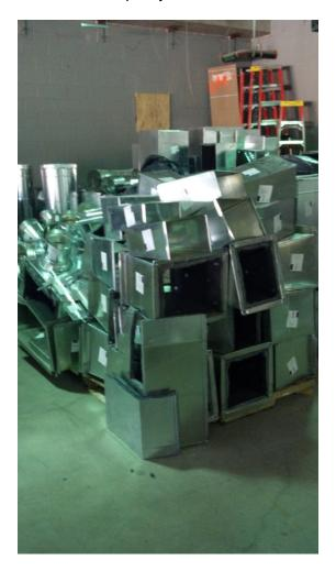
2) Recommend covering inlets and outlets of FPVAV boxes to prevent dust from getting on the coils or in flow crosses and ensure future indoor air quality.
